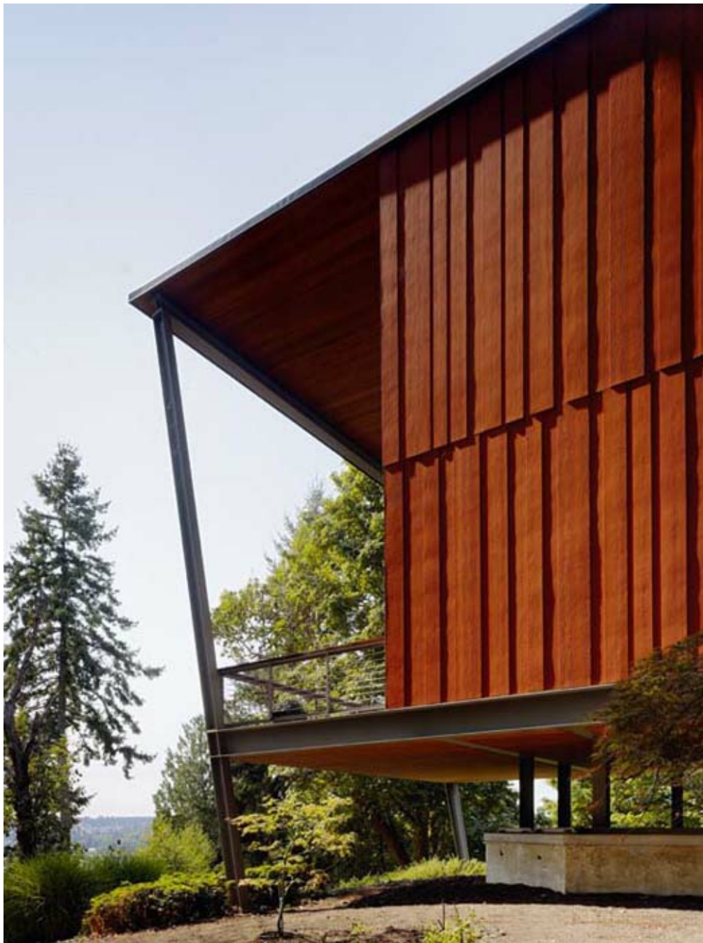
A tilted steel brace holds up the sharply canted roof.
