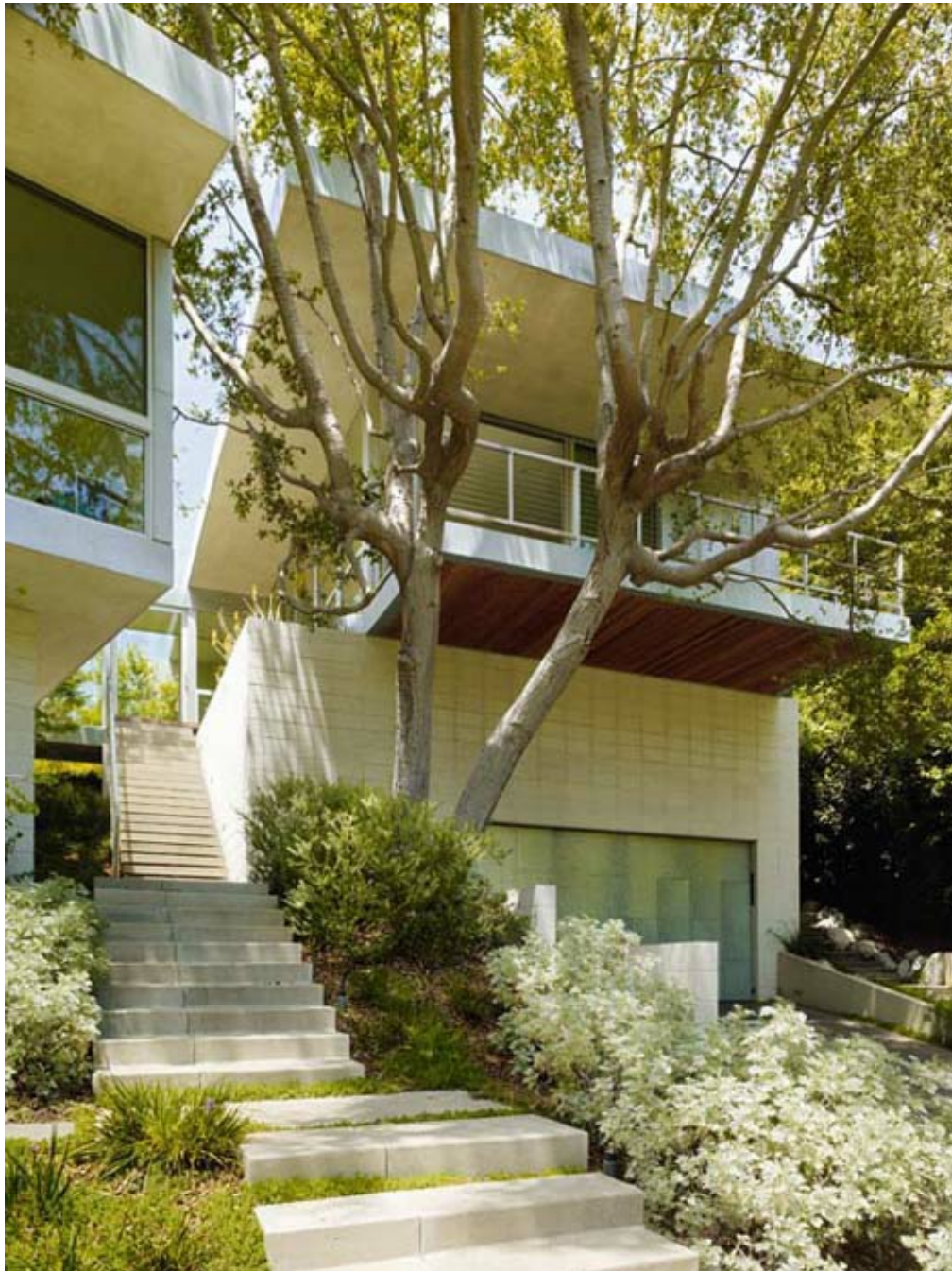
Above and Below: At the top of a curved driveway, burnished concrete block basements contain a garage and, on the
