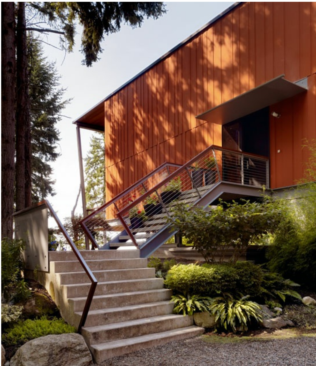
A galvanized steel and concrete front entry stair on the east side is weather resistant.
