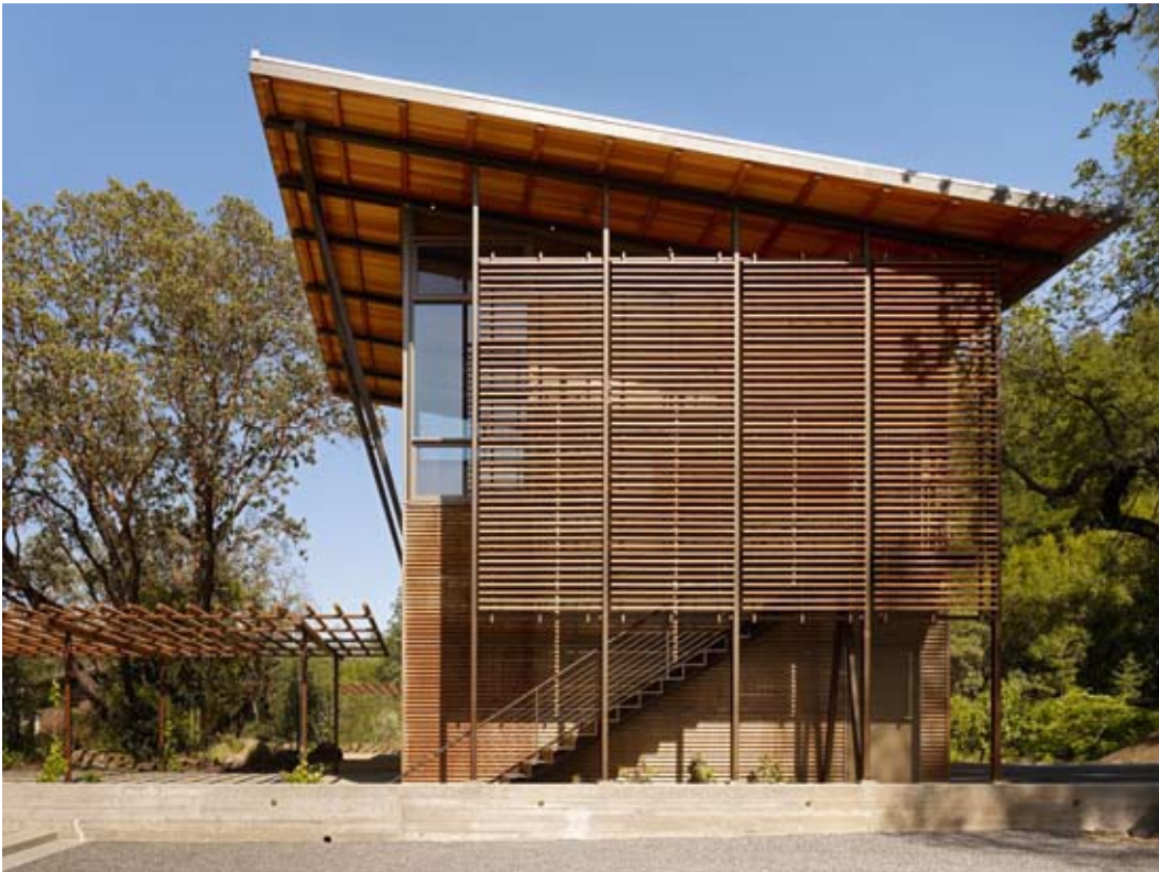
Above and Below: The children’s pavilion has stairs shaded by a slatted wood screen.
