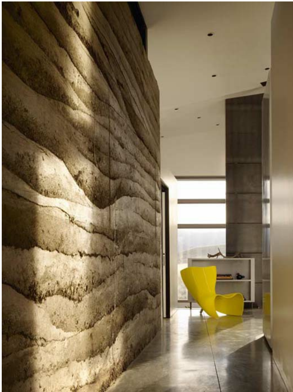
The earth for the wall came from the site. The Felt chair is by Marc Newson.
