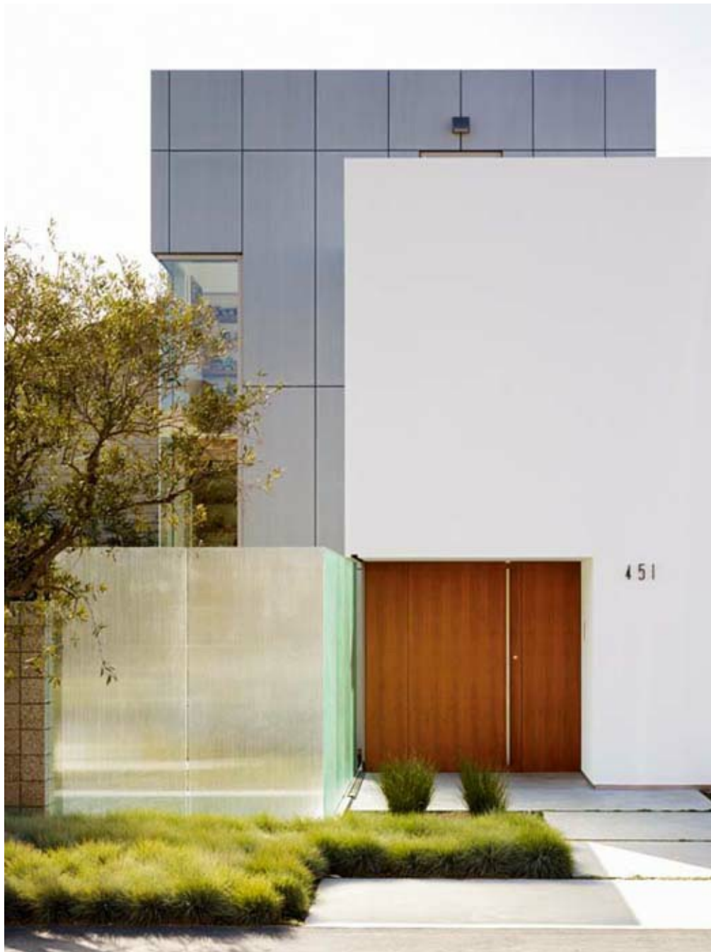
The front door; RHEINZINK panels cover the stair tower.
