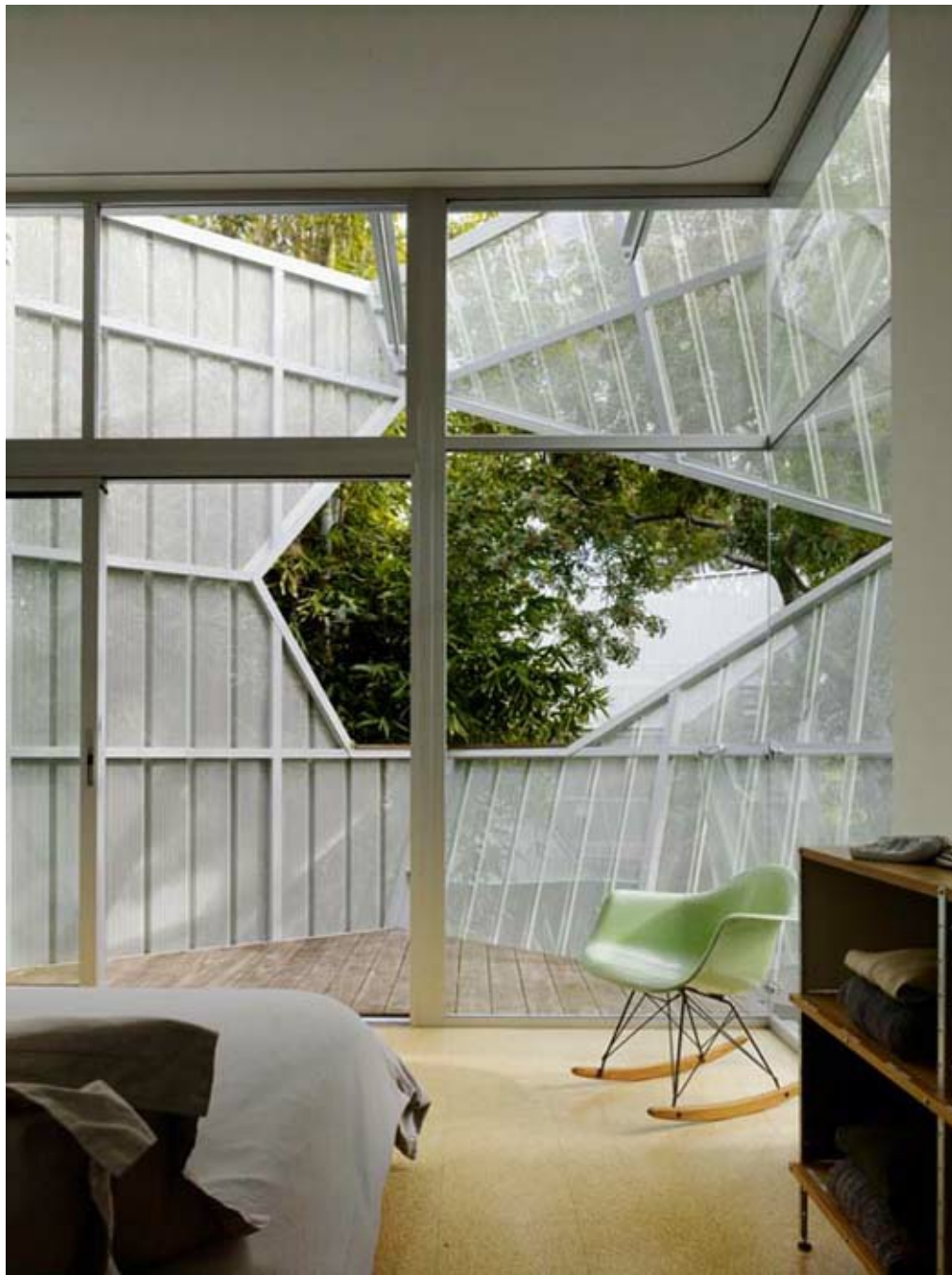
Doors slide open for ventilation. Strategic openings in the mesh let in light, yet afford ample privacy. The molded fiberglass rocker is by Ray and Charles Eames.
