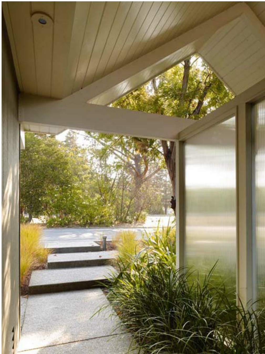
Under the peaked section of the roof, the entryway and an atrium share fritted glass panel walls.
